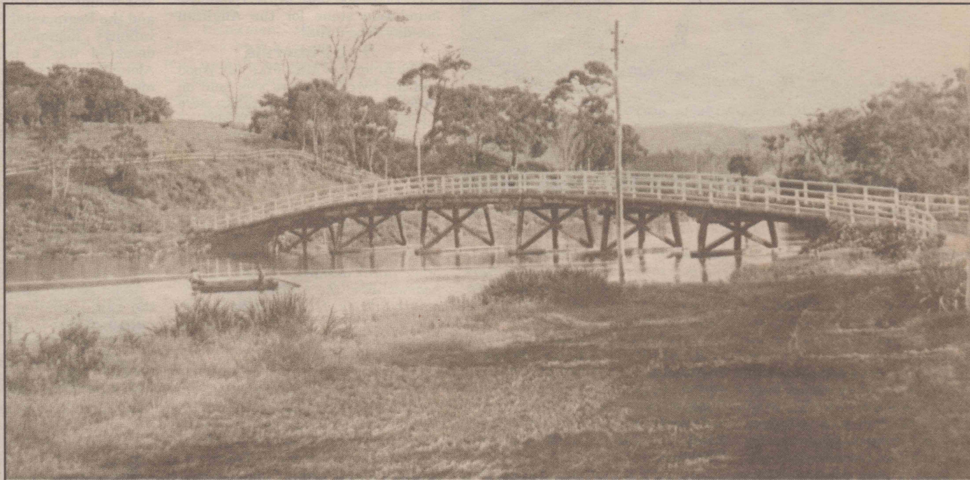
The first Minnamurra Bridge - a timber, one-lane thoroughfare built in 1870 by Shellharbour Council at a cost of £1000.
