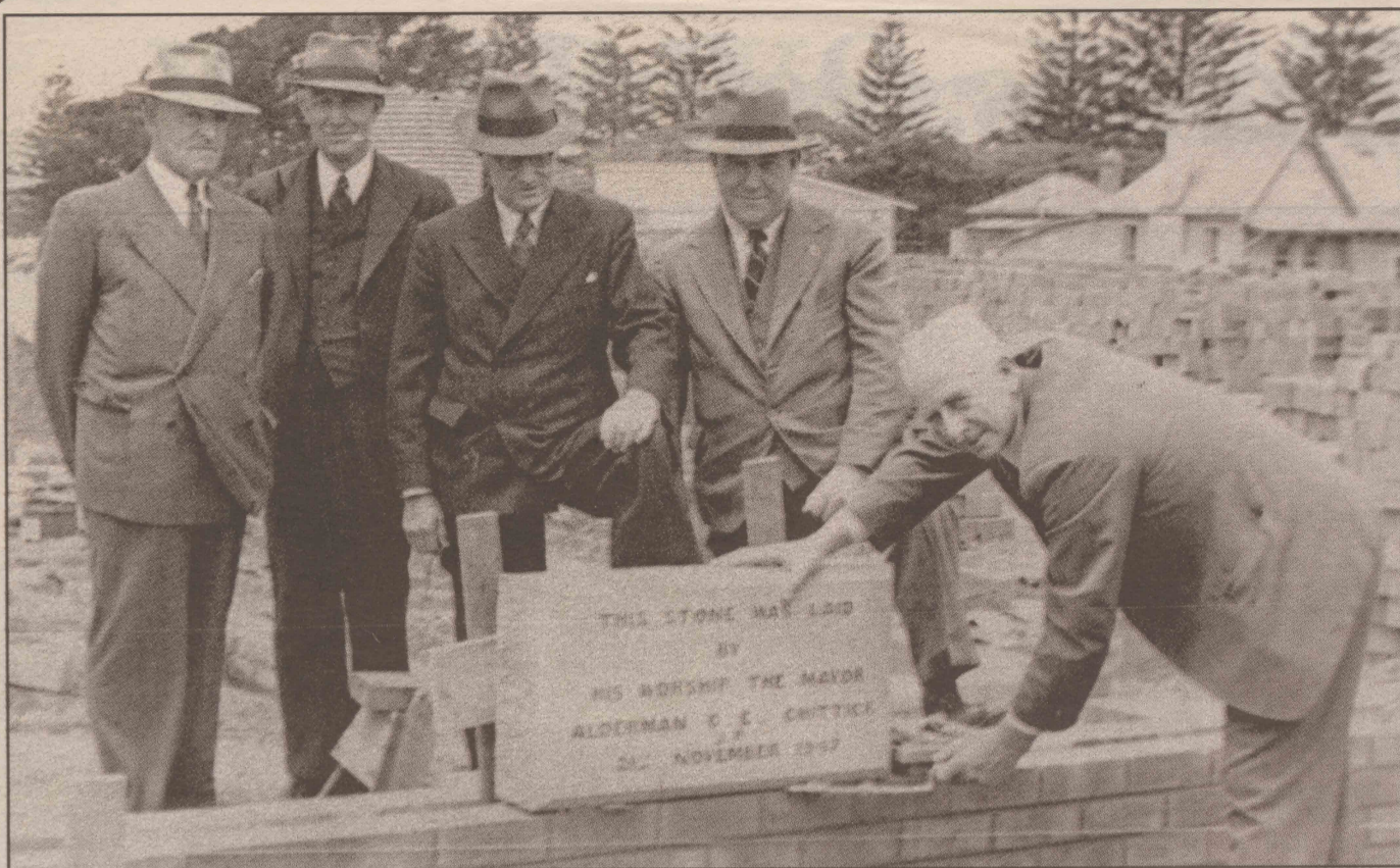
Gerringong Mayor, Ald Mayor Gus Chittick, lays the foundation stone for the new Gerringong Town Hall watched by (from left) CT Hindmarsh, JRM Miller, architect Ray Spencer and HG Miller.
