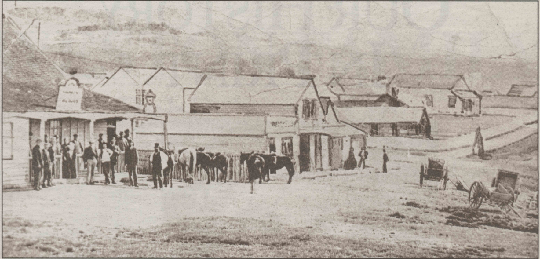
• This is believed to be the earliest photo of Terralong Street - circa 1860. It shows the Steam Packet Hotel and Cook's Blacksmiths Shop. The long slab shed to the right is the early Show Pavilion and beside that is the original Kiama Courthouse. A new courthouse was built in its place in 1861.
